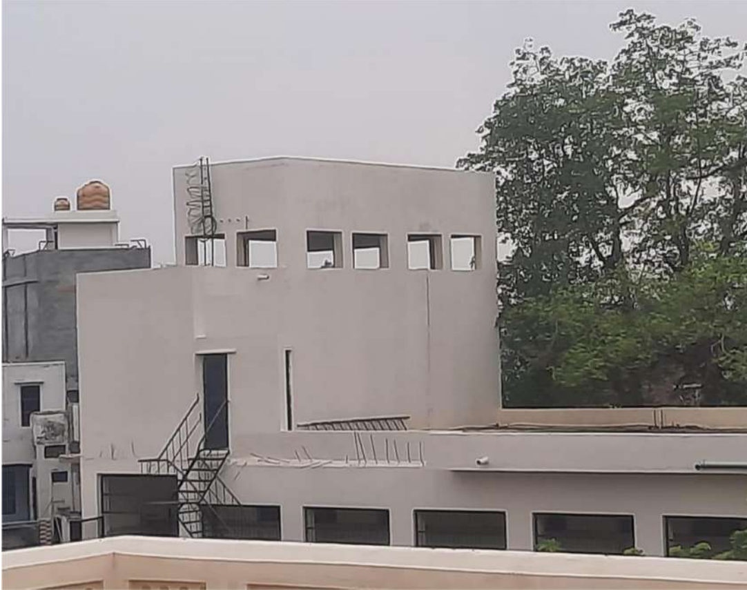
Drinking Water storage tank
