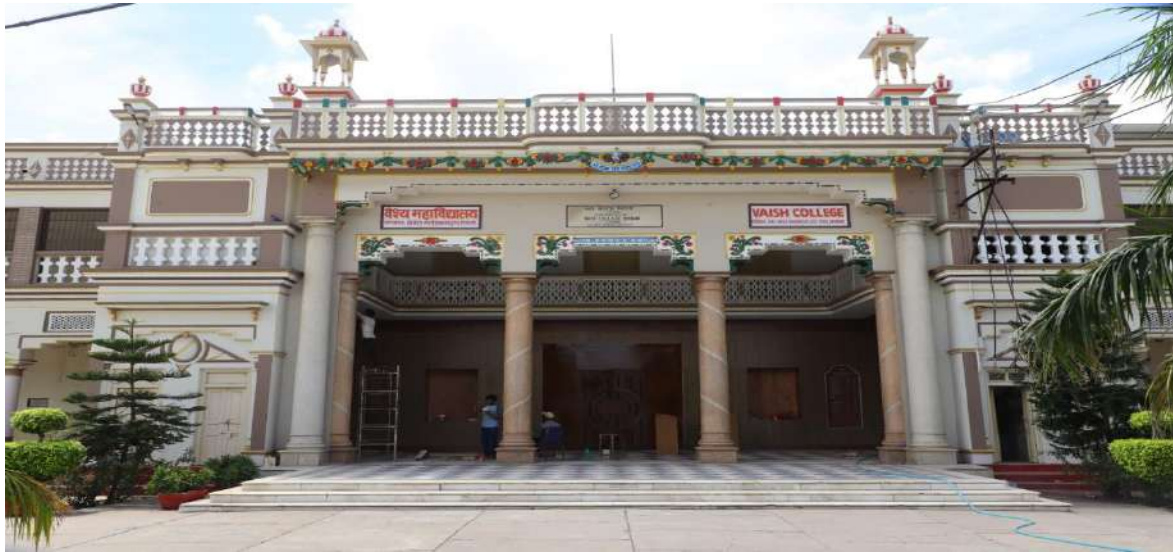
COLLEGE AUDITORIUM OUTSIDE VIEW
